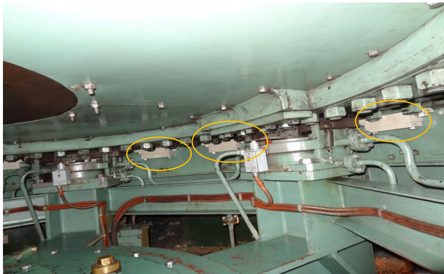
Fig. 9 Balancing weights under the generator (in the LGB zone)
