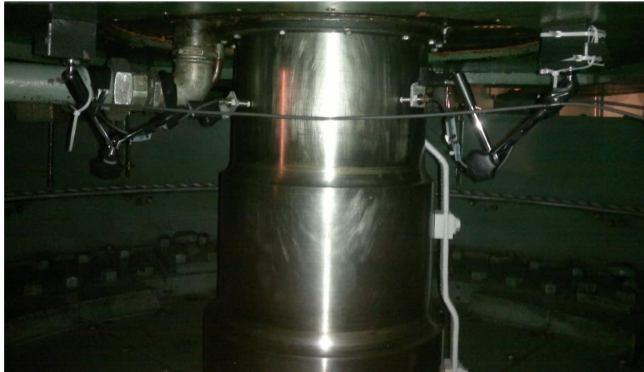
Fig. 4 Sensors under UGB (and under the thrust collar).
